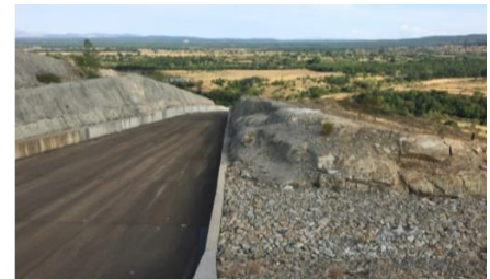
(c) View of the dam spillway
