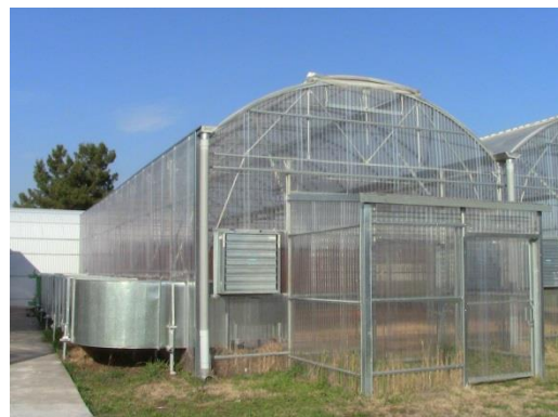
Picture 3. South side view of the prototype greenhouse located in Larissa, with the rectangular isolated duct of the water/air recycling unit.
