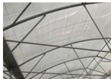
Figure 7 Representative photos of the gothic greenhouse structure in Central Greece
